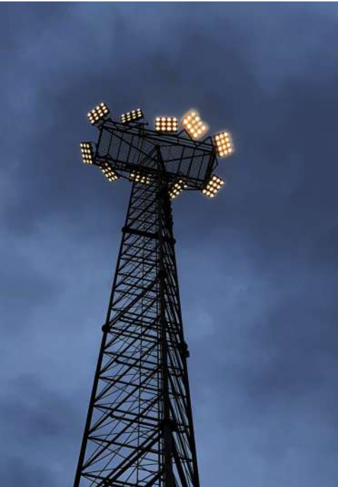
Belgian Dock LED Lighting Project ▼
