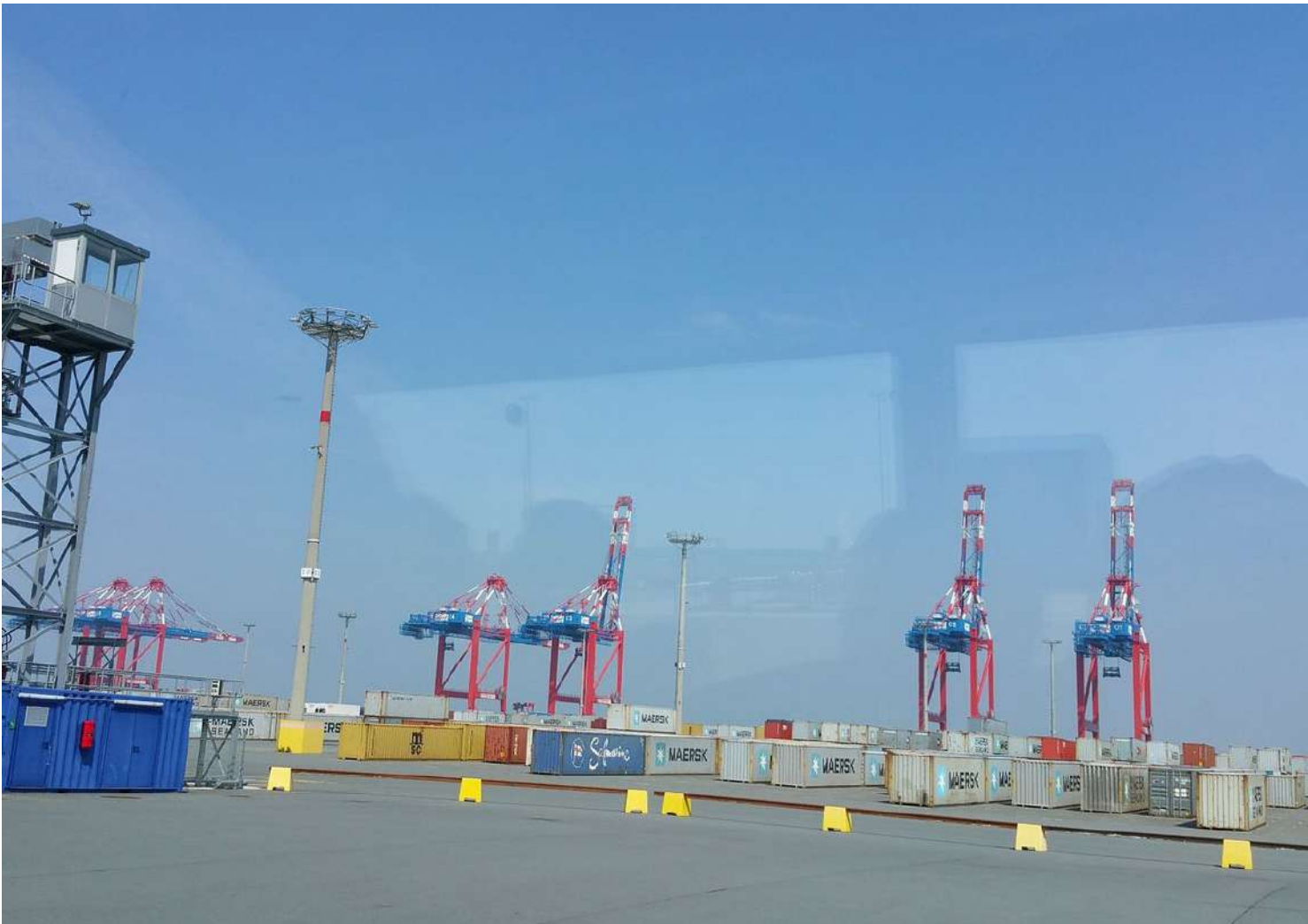
German Port LED Lighting Project ▲
