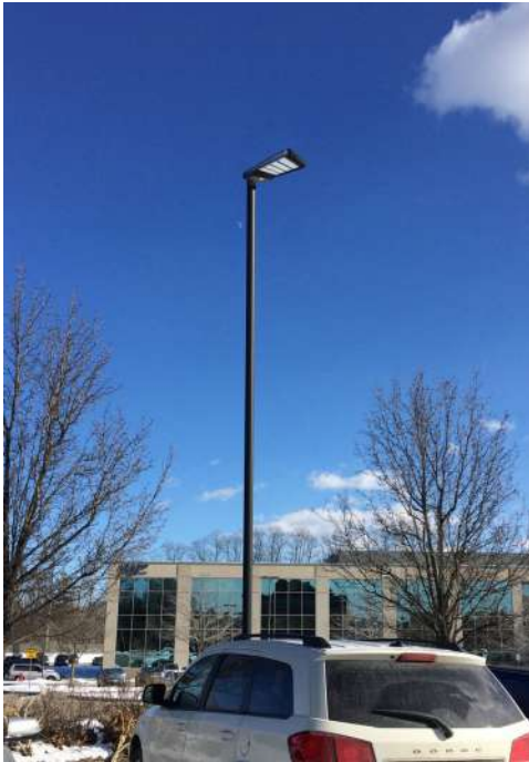
American LED Street Light Lighting Project ▼
